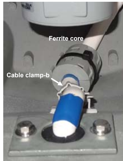
14) Clamp the cable by the cable clamp-b.
